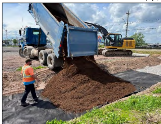
Bioswale #2 - Construction (left) of the bioswale and finished project (right)
