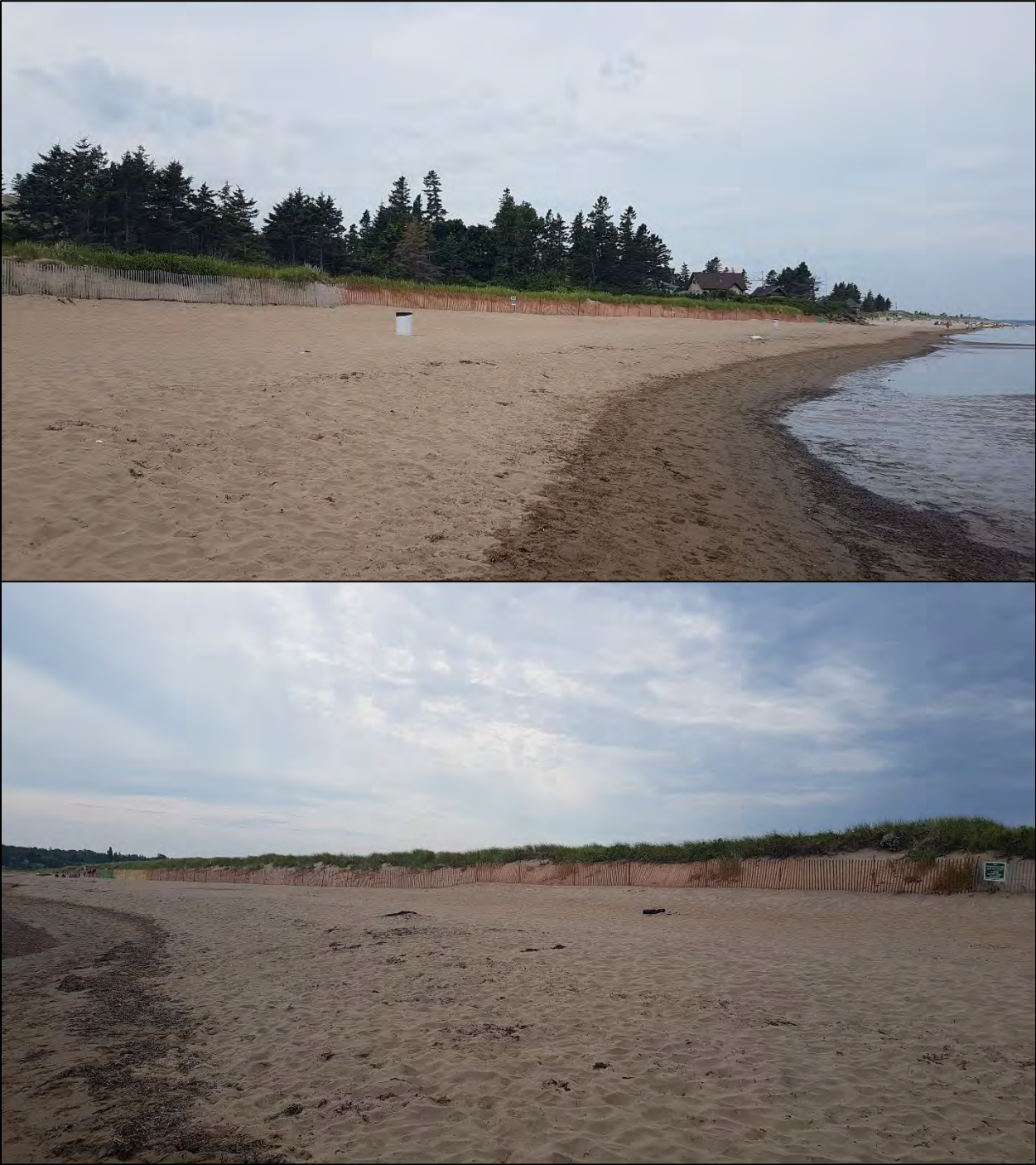
Figure 38: Dune fencing installed at Belliveau beach (Top & Bottom)
