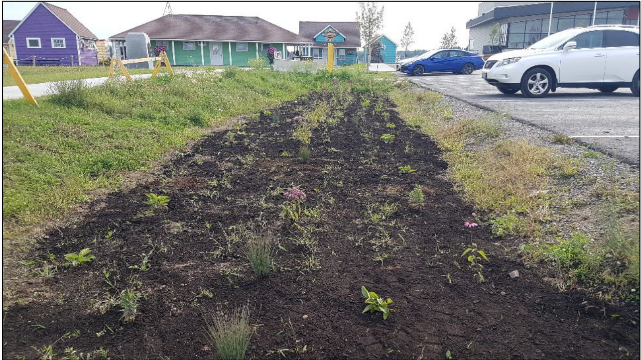
Figure 6. Homarus Centre Bioswale #2 Construction (Part 2)
