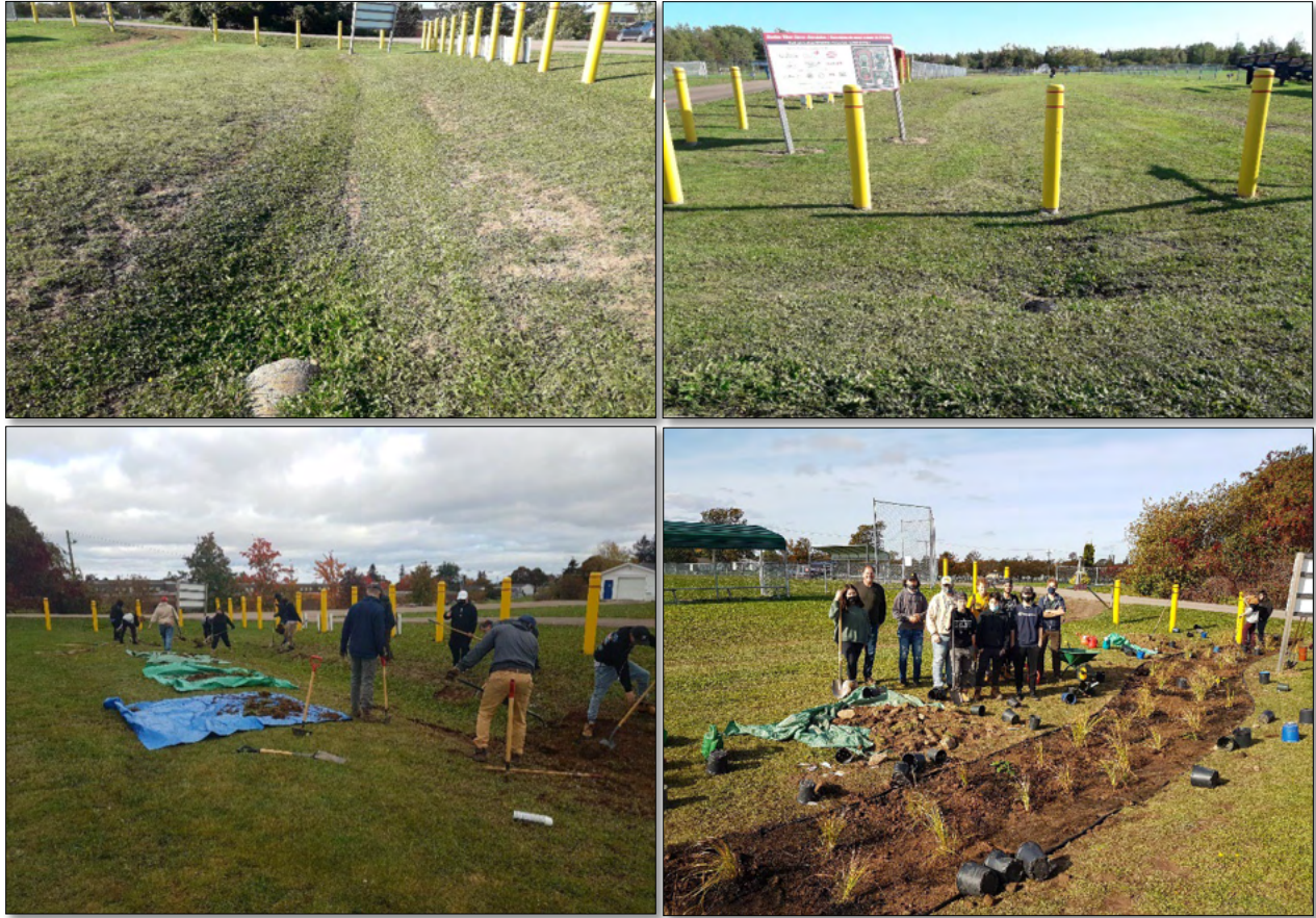
Figure 14: Before photos and construction of the L.-J.-R bioswale (2021)
