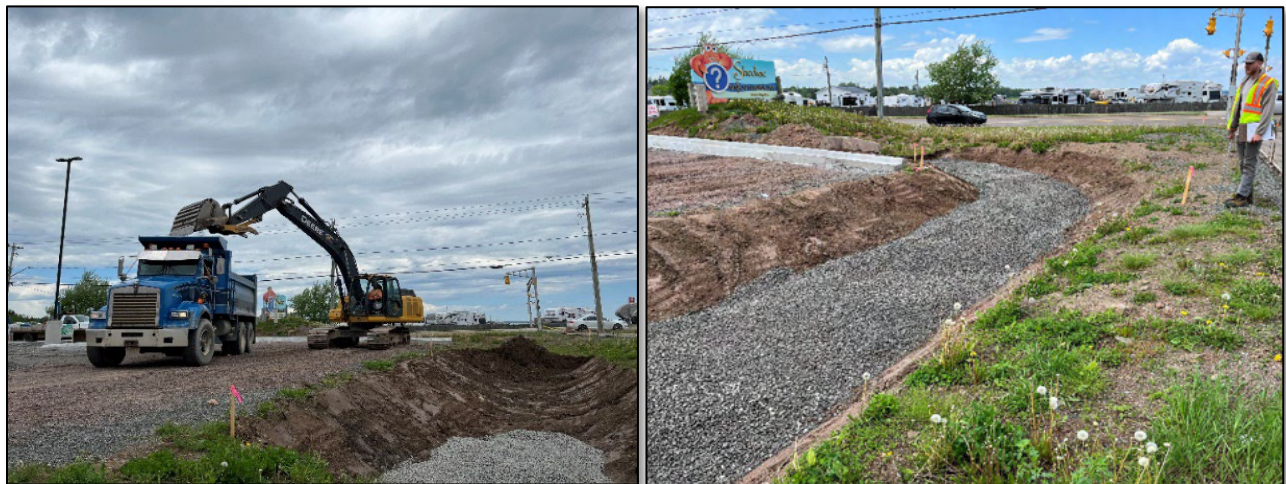
Figure 5: Homarus Centre Bioswale #2 Construction (Part 1)
