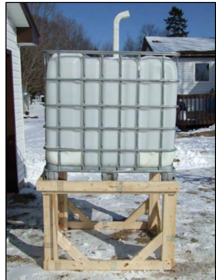
Figure 22: Example of a RWHS using a 1,000 L tote Source: EcoContainer Co. Facebook Page
