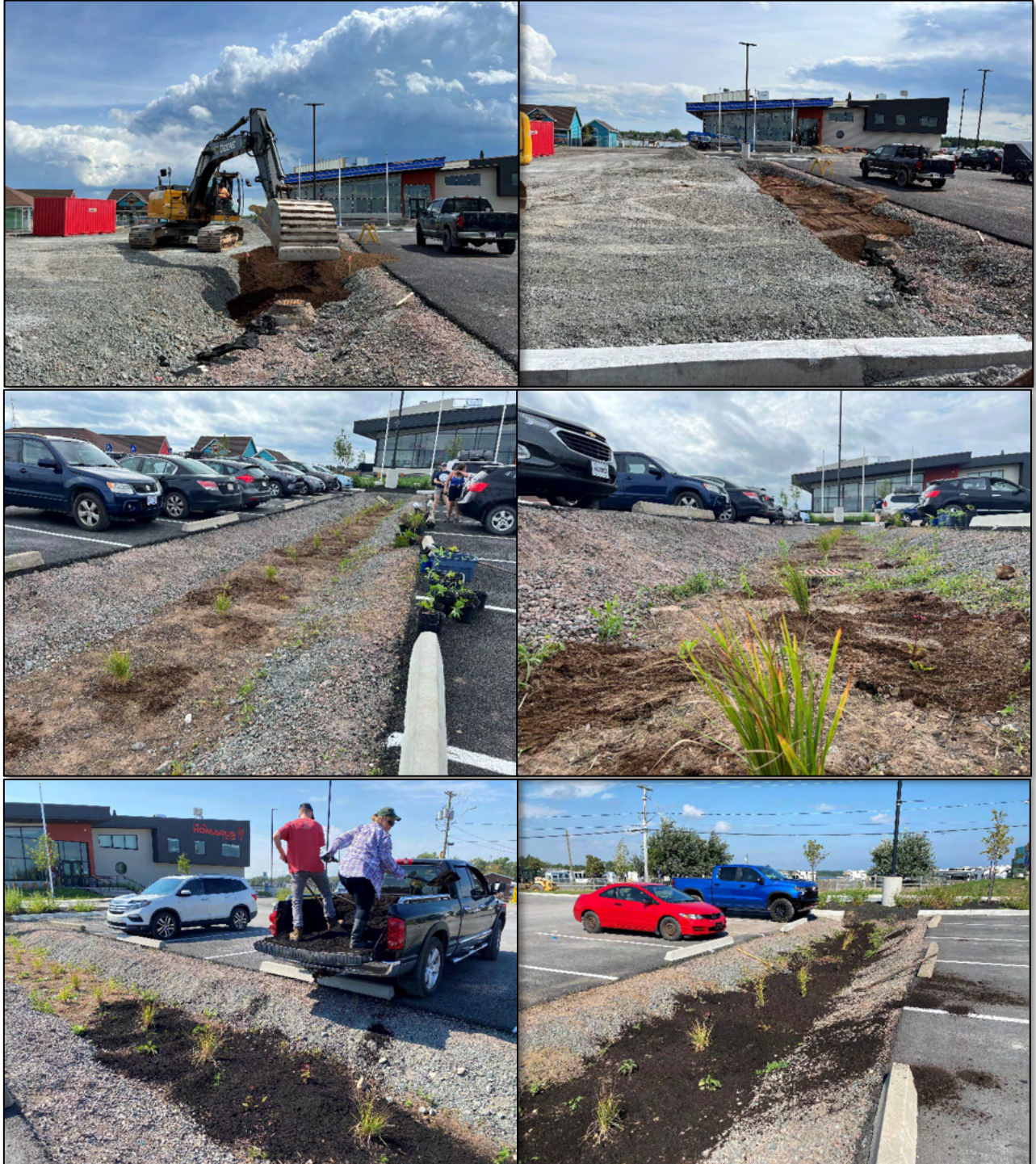
Figure 7. Homarus Centre Bioswale #1 Construction
