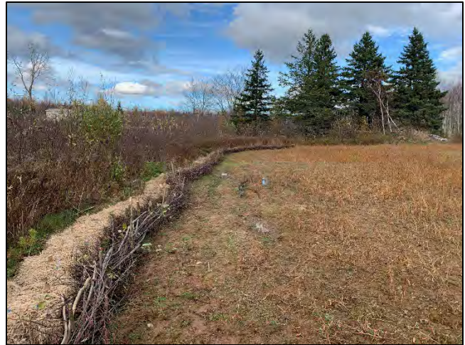
Figure 41: Staked haybales and wattle fencing.
