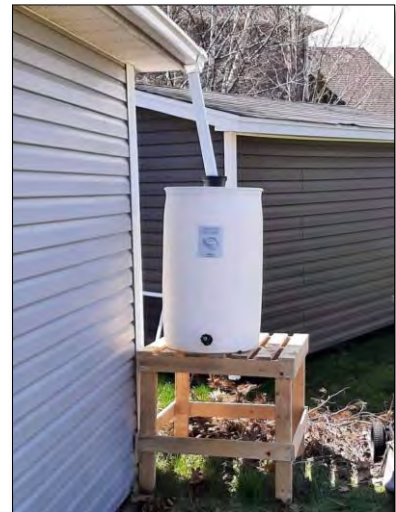
Installed rain barrel
