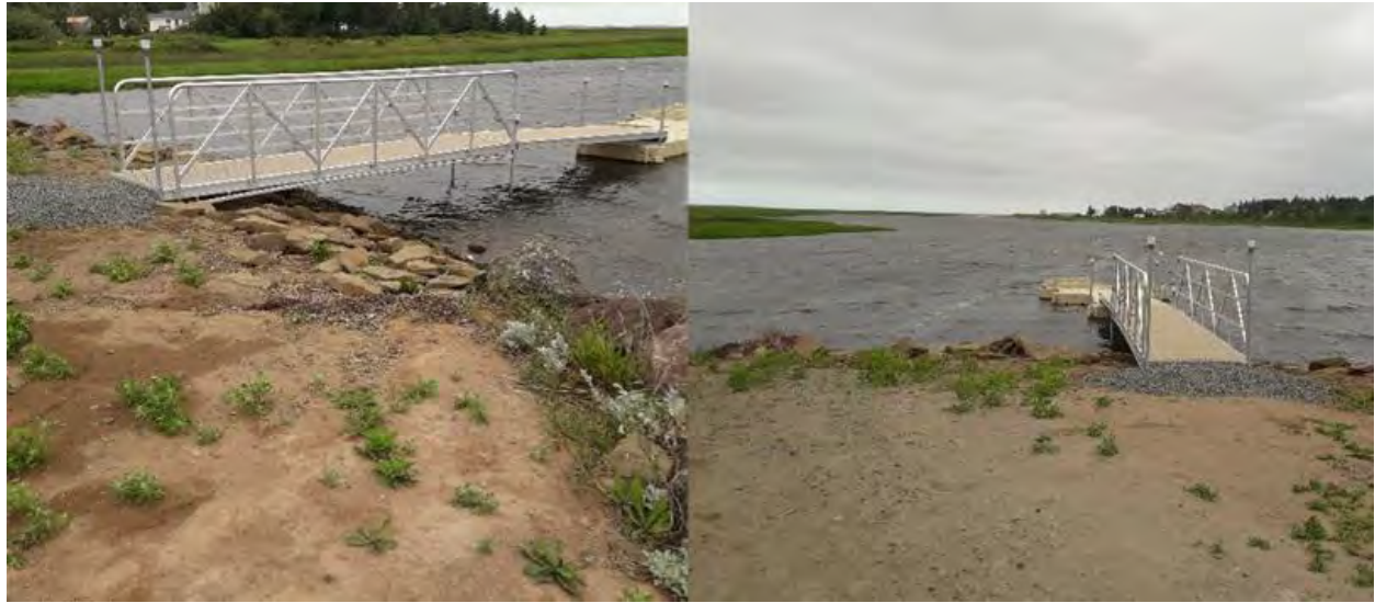
Figure 33: Before photos of the dock area of the restoration site in 2019
