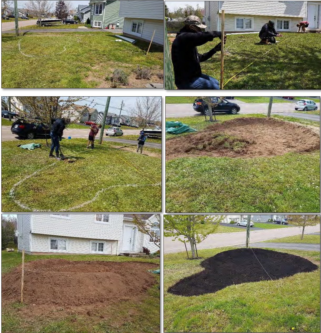
Figure 15: Rue Rachel rain garden under construction
