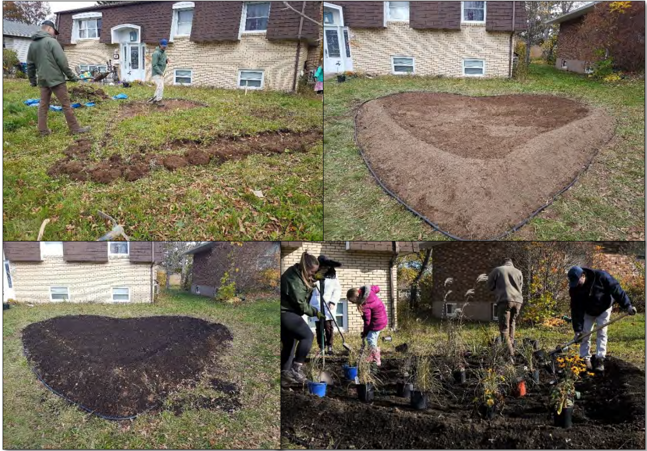
Figure 19: Rue. Smith rain garden under construction
