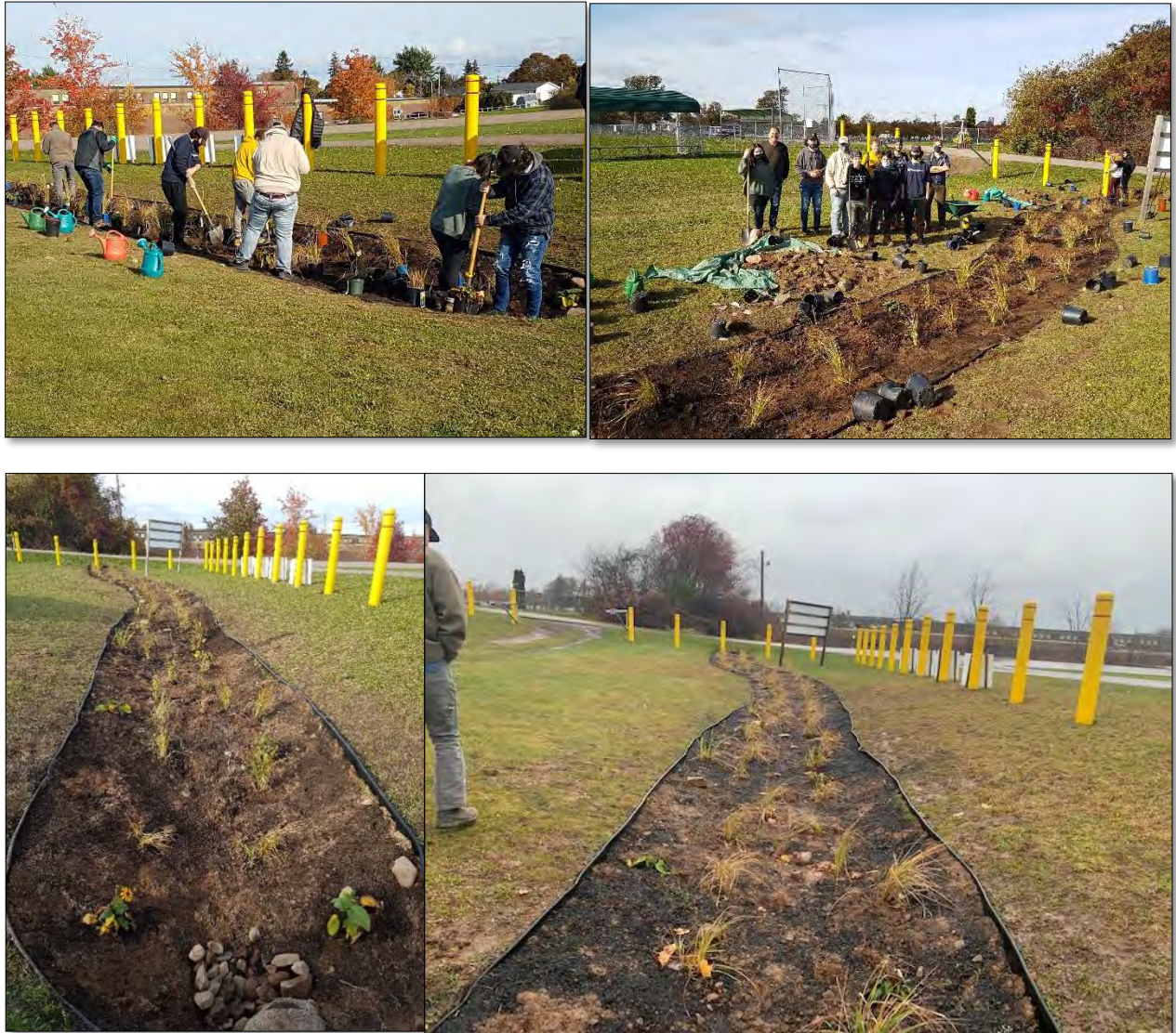
Figure 6: LJR bioswale completed
