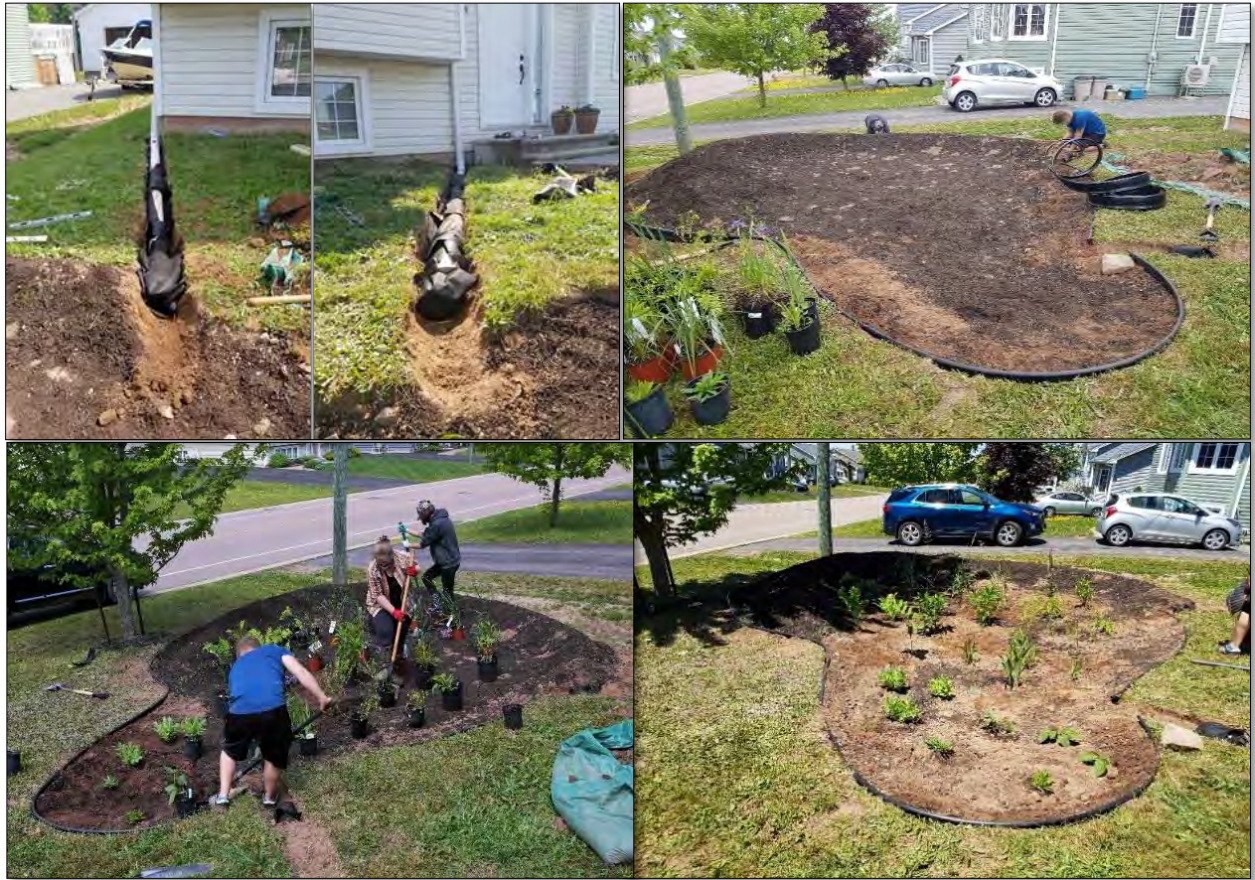
Figure 16: Rue Rachel rain garden under construction
