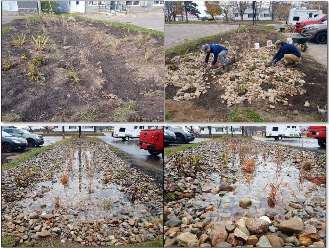
Figure 13: Completed bioswale at Maximum Signs & Time2Shine after rainfall event
