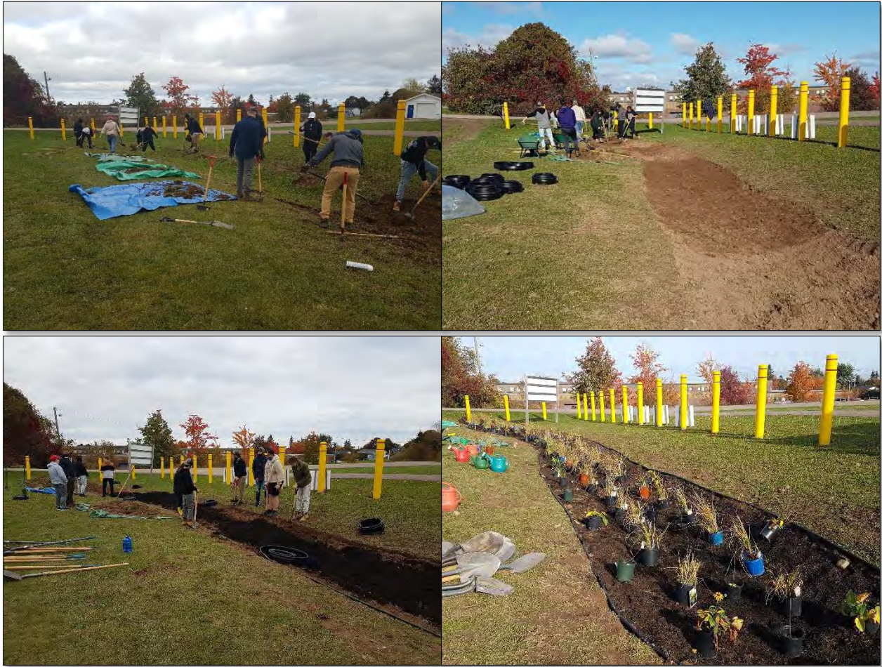
Figure 5: LJR bioswale under construction with students
