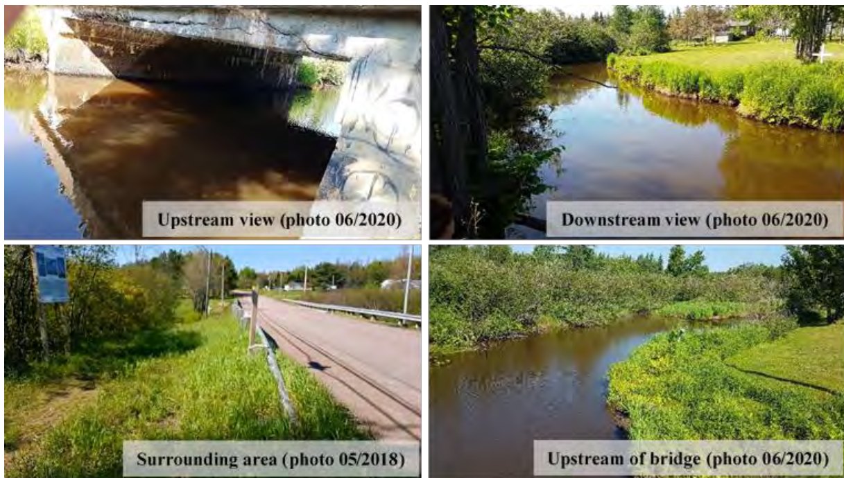
Figure 18: Site photos for water quality sampling site ScdB
