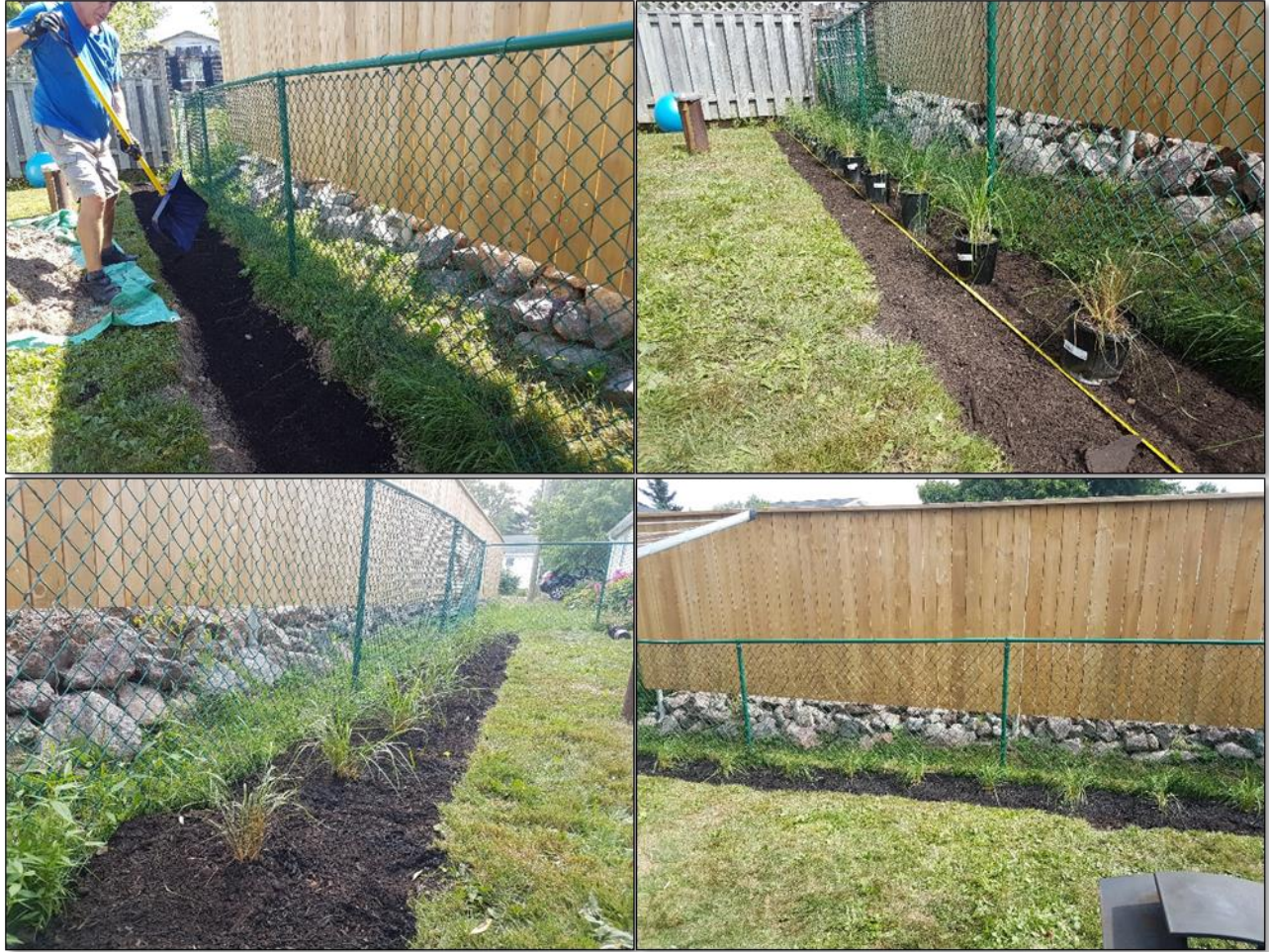
Figure 13: Residential Bioswale #1 – Construction Photos Part 2 (August 2020)
