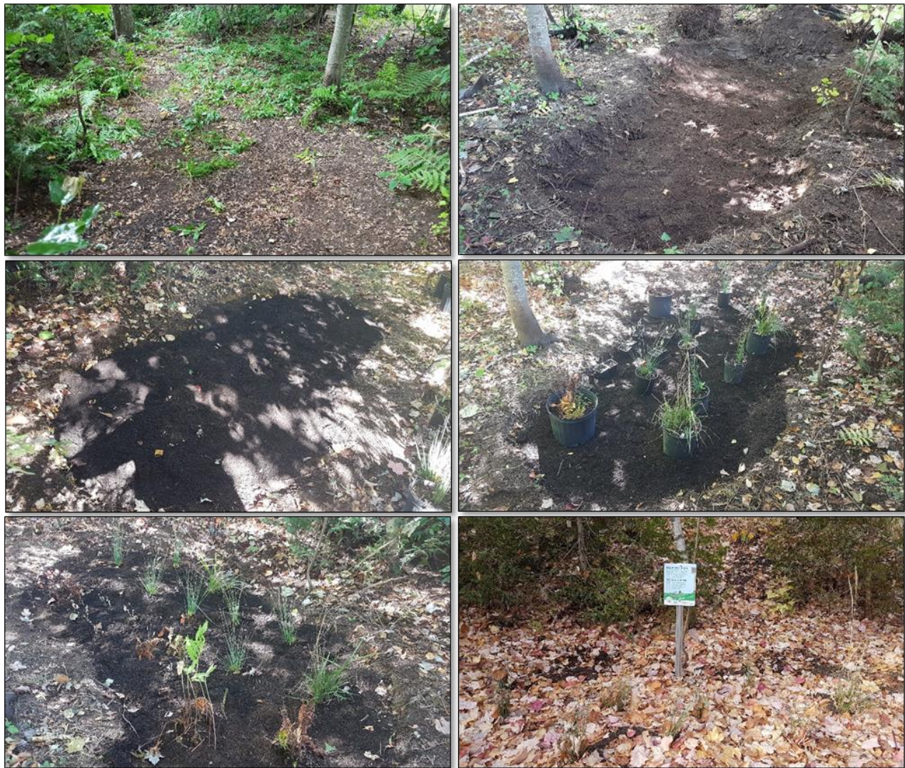
Figure 18: Residential Rain Garden #3 – Construction Photos (September 2020)
