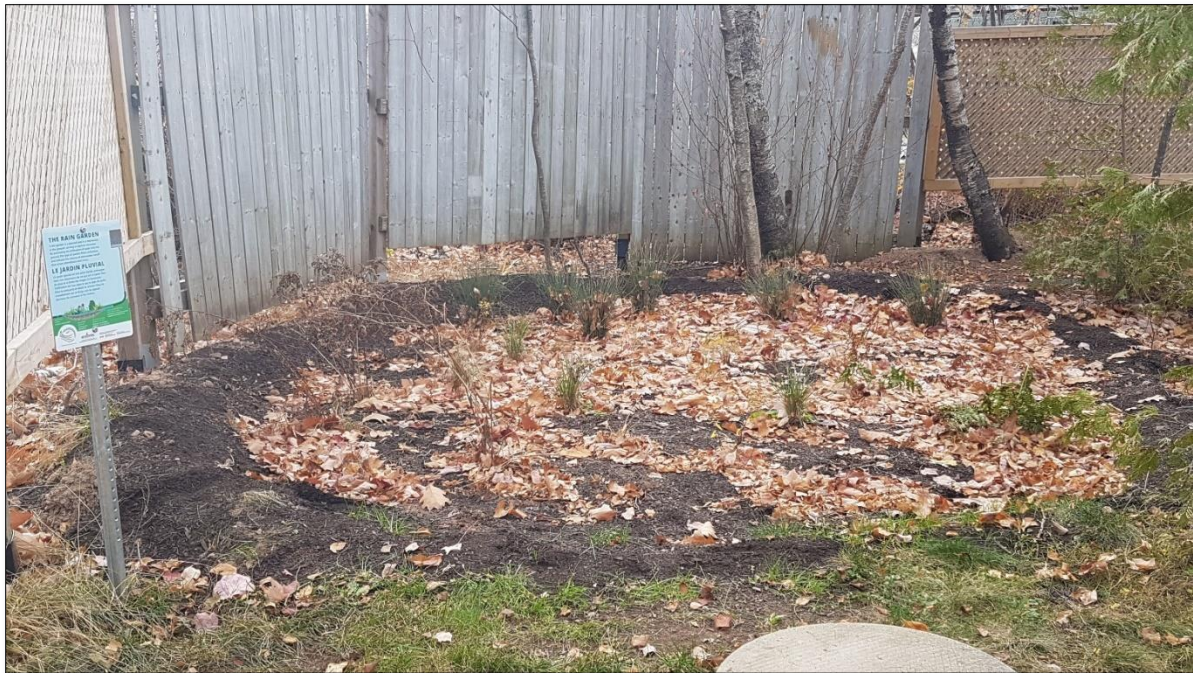
Figure 17: Residential Rain Garden #2 – Sign Installation (October 2020)
