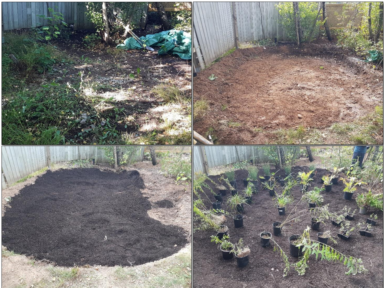
Figure 15: Residential Rain Garden #2 – Construction Photos (September 2020)
