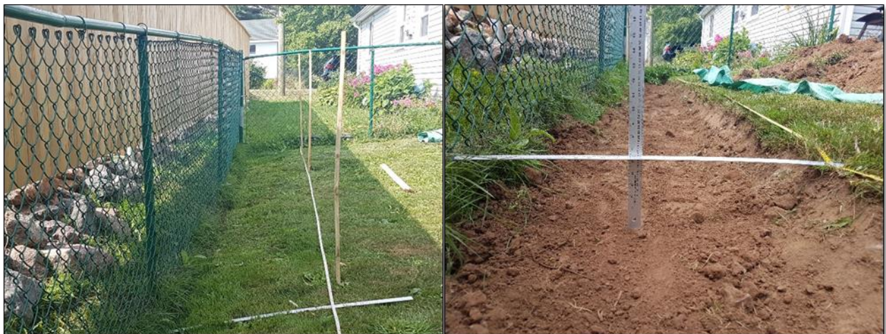
Figure 12: Residential Bioswale #1 – Construction Photos Part 1 (August 2020)
