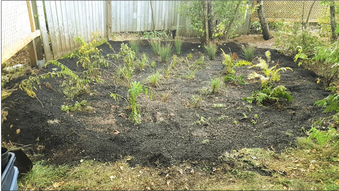
Figure 16: Residential Rain Garden #2 – Completed (September 2020)
