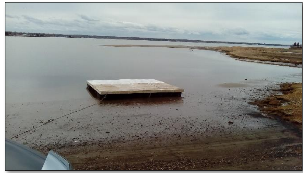
Figure 14: Sections being towed from marina to work site beside walking trail
