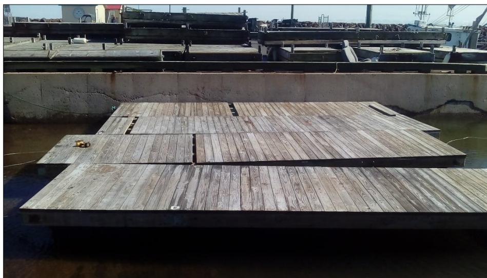
Figure 13: Nesting platform sections floating before being attached together as one unit
