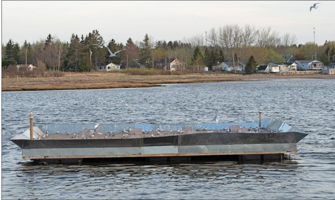
Figure 5: New platform built in 2020
