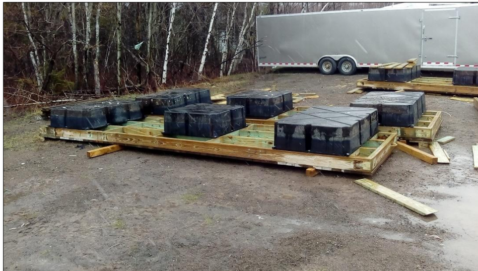
Figure 12: Sections being rebuilt to produce a new nesting platform 2020
