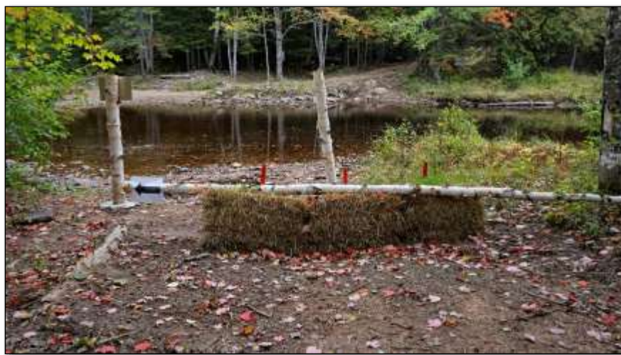
Figure 13: ATV access blockage and sediment control (hay-bale check dam)
