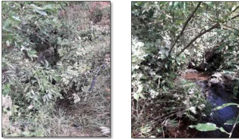
Figure 40: Before and after photos of the shrub thinning upstream of the culvert
