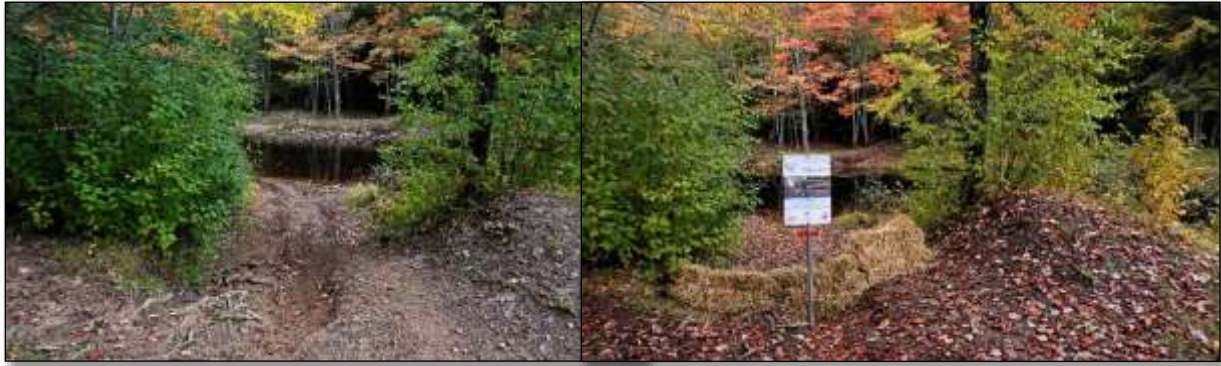
Figure 36: Before and after photos of ATV access blockage and sediment control (hay-bale check dam)
