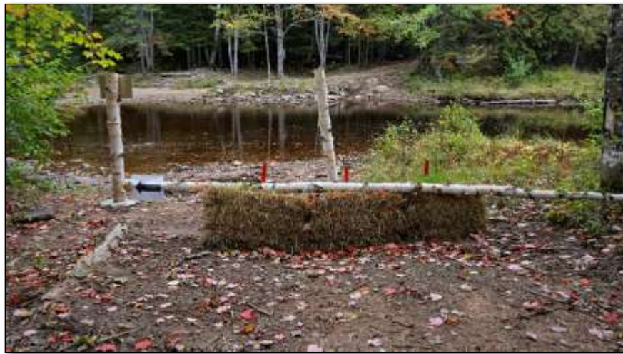
Figure 37: ATV access blockage and sediment control (hay-bale check dam)
