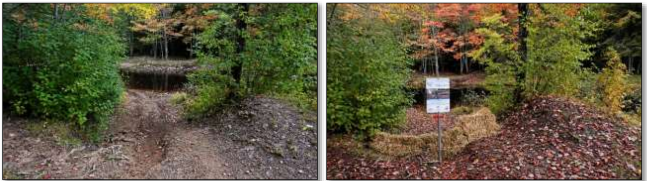
Figure 22: Before and after photos of ATV access blockage and sediment control (hay-bale check dam)
