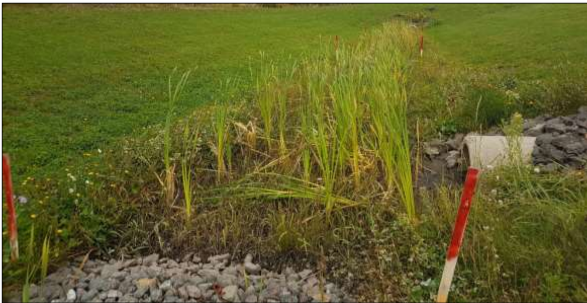
Figure 10: Photo of bioswale growth in the fall of 2019
