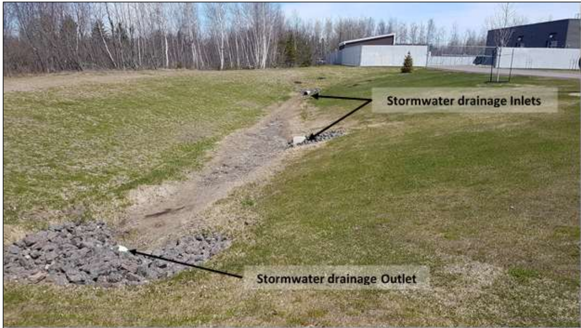
Figure 3: Stormwater basin – drainage inlets and outlet
