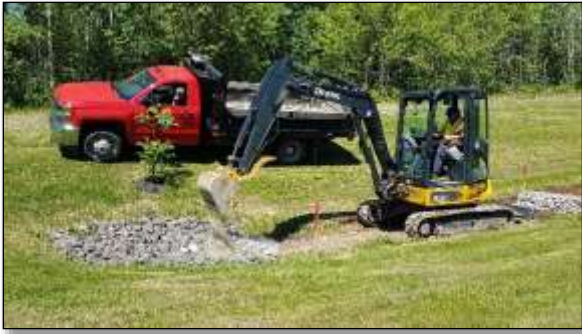
Figure 7: Installation of rocks, check dams and top soil
