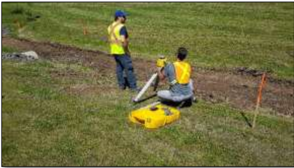
Figure 6: Elevation measurements taken by Luko Construction for check dam installations
