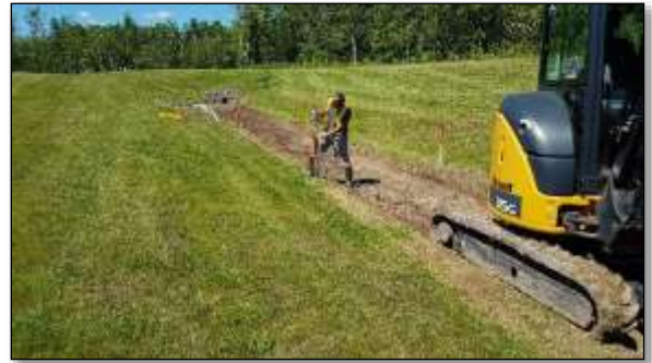
Figure 6: Elevation measurements taken by Luko Construction for check dam installations
