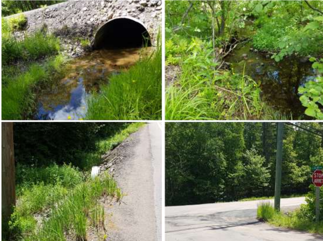
Figure 14: Site photos for the water quality monitoring station WQ-6
