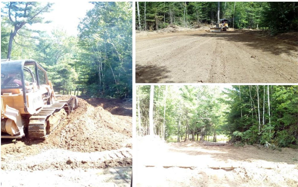
Figure 19: Work photos of machinery on the ATV trail, Scoudouc River 2017
