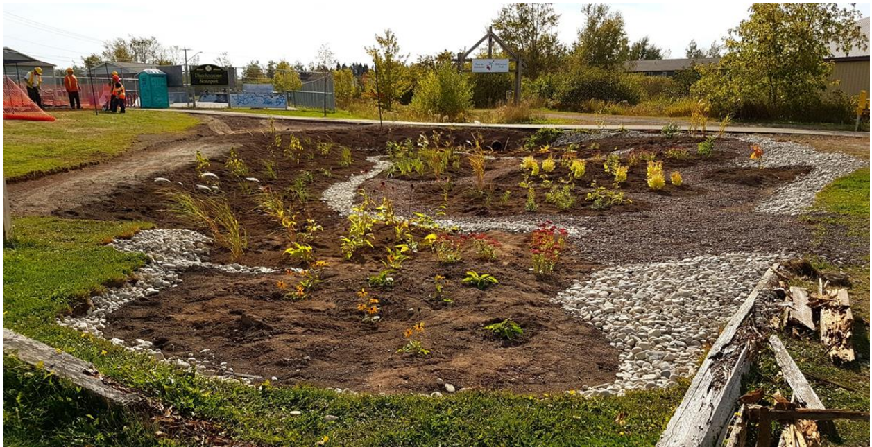
Figure 29: Rain garden construction photos, 2017
